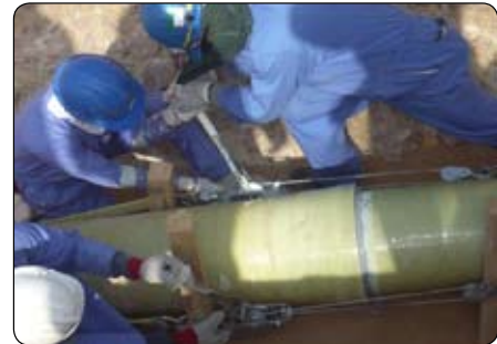
Assembly of a Joint Using Mechanical Pullers
