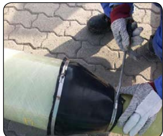
Tightening the endseal with juggle clamp
