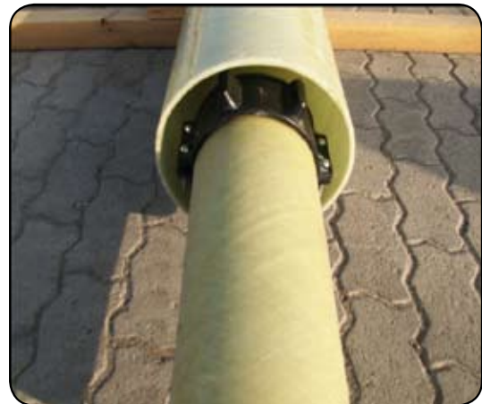
Pipe fixed with centralizer inserting inside the casing
