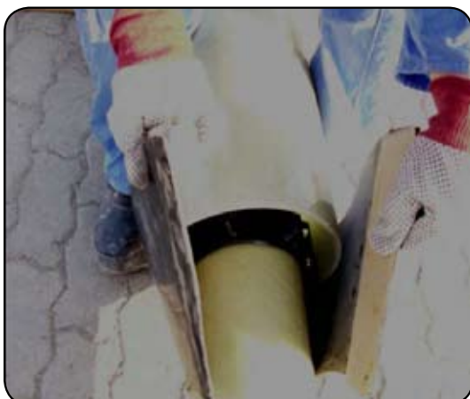
Fixing of End Seal
