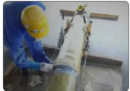
Assembly of a Joint Using Mechanical Pullers
